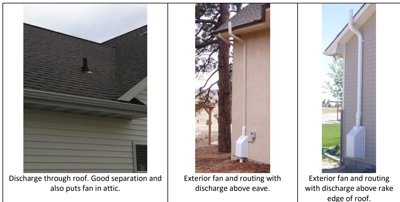
Figure 66: Proper Discharge Points
