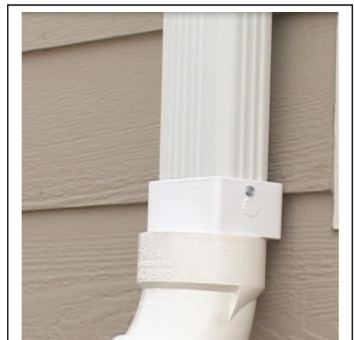
Figure 63: Adapting exterior pipe to downspout
