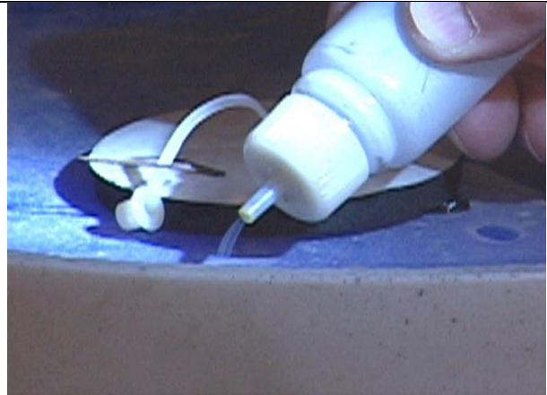
Lids on sumps to which a radon system is connected can leak significant amounts of air. This should be gasketed and bolted.
