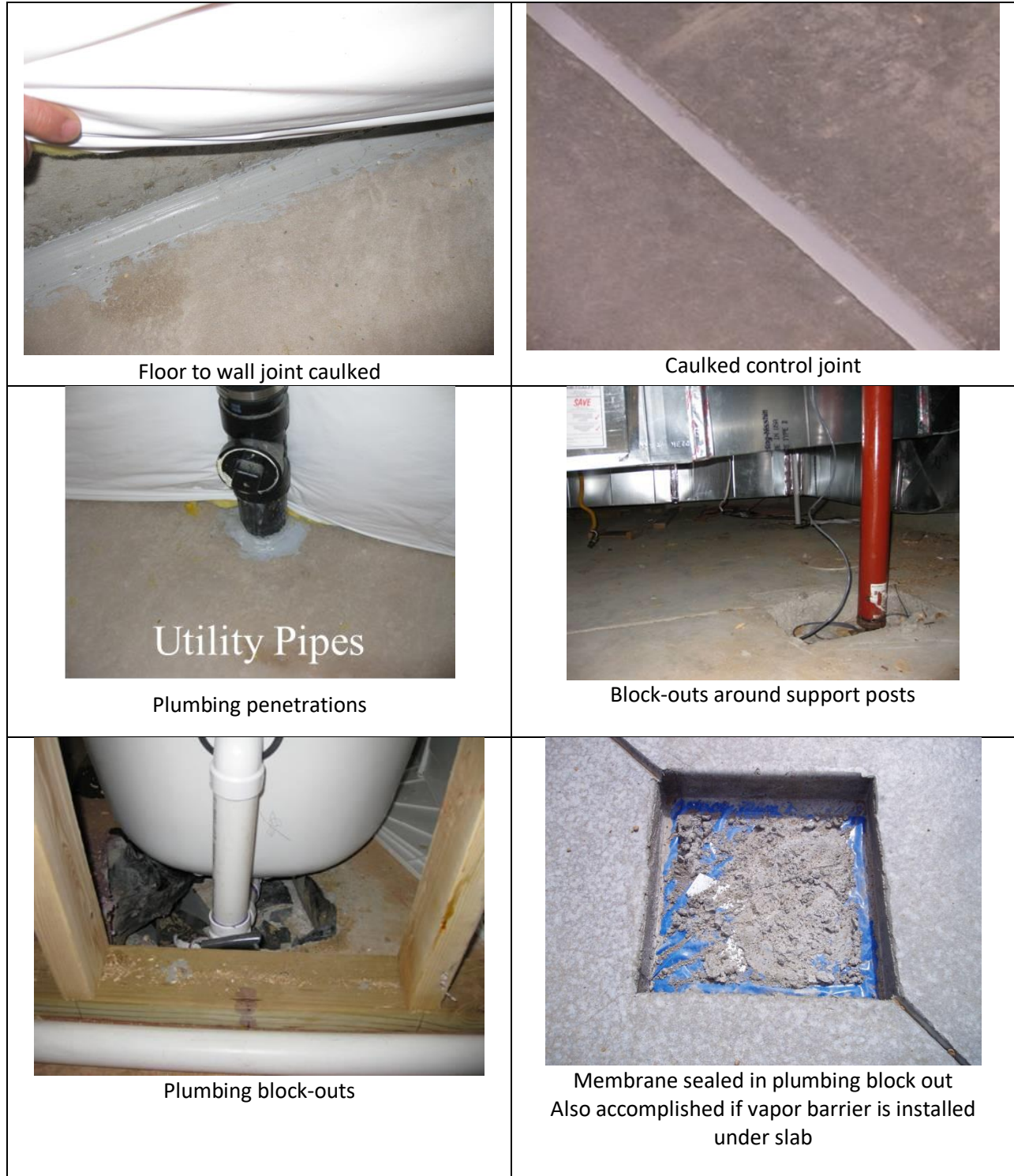
Figure 75: Slab Caulking and Sealing Examples
