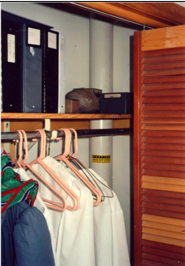
Interior routing hides system routed up through closets
